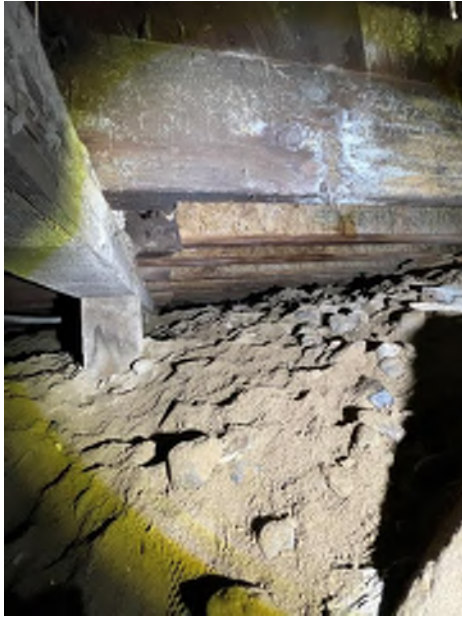
Photo No. 1 (Crawlspace post on dirt)
