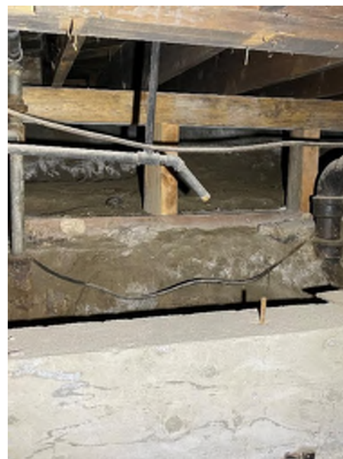
Photo No.4 (Timber footings on dirt)
