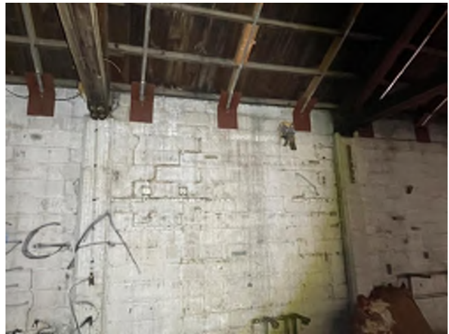
Photo #8 (Rafter to wall seismic ties)
