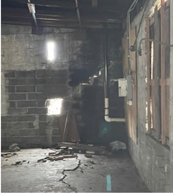
Photo #1 (Cracked/ separated Wall, east side)
