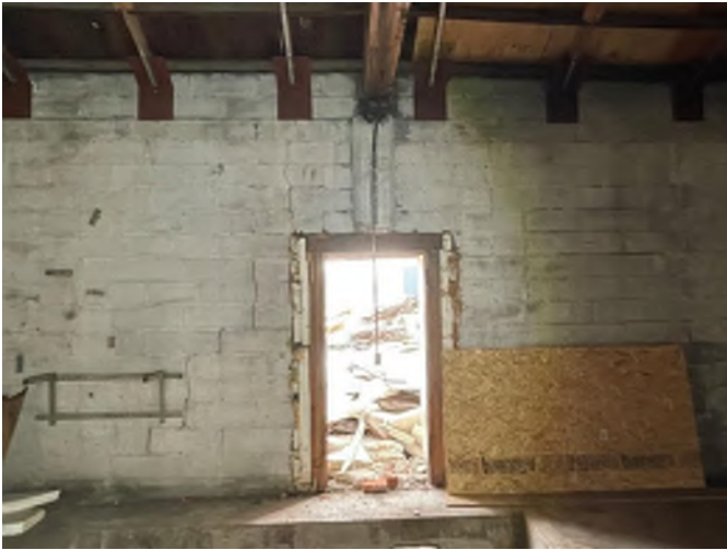
Photo #5 (Door through pilaster)
